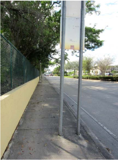
Observed sidewalk obstructions include utility poles in the middle of the sidewalk, with additional cables blocking the path for an alternate route (Top Left, Image source – Google Earth), Utility boxes and fire hydrants in sidewalks (Top Right), traffic signs (Bottom Left), and fire hydrants in sidewalks at curb areas (Bottom Right), all of which present issues for pedestrians, and some of which are non ADA compliant.
