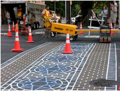
Painted/textured crosswalks can be achieved through the application of thermoplastic striping, and applied to raised crosswalks as well.
