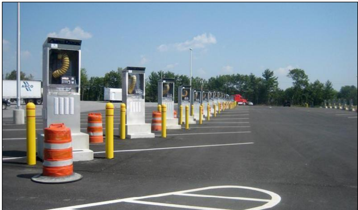
Airedock Pedestal Truck Electrification System
