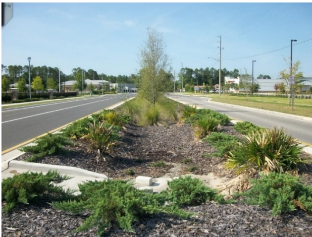
Figure 54: Green Infrastructure Examples in Florida: Low Impact Design, Bioswales & Raingardens
