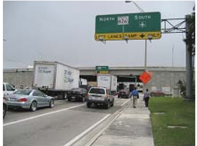
NW 25th Street at Palmetto Expressway
