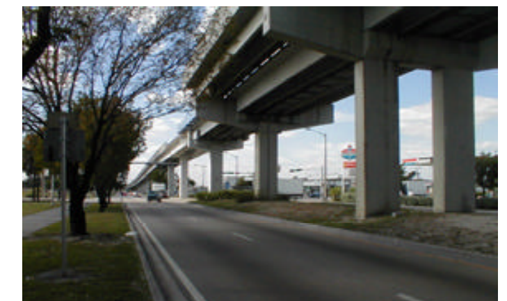
Westbound NW 79th Street
