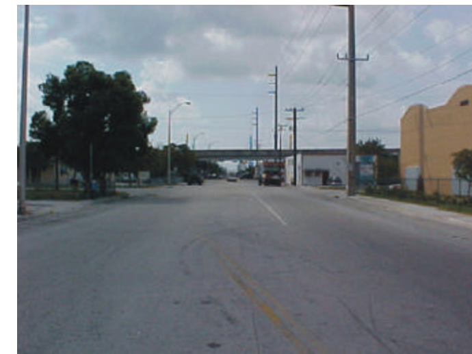
Existing NW 37th Ave. Looking South
