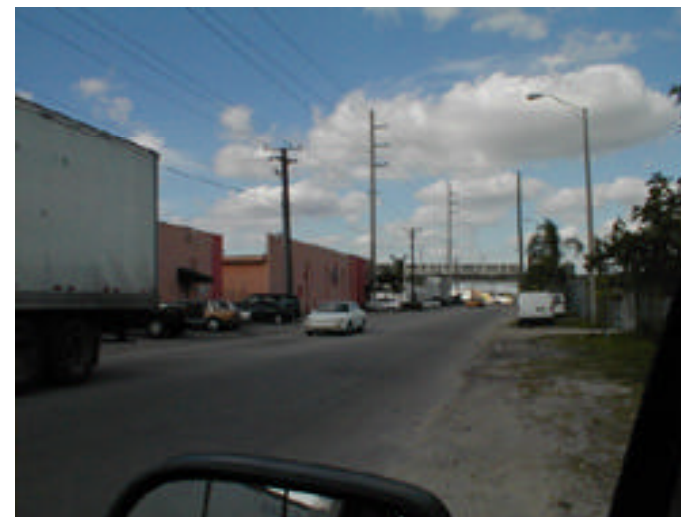
Existing NW 37th Ave. Looking North
