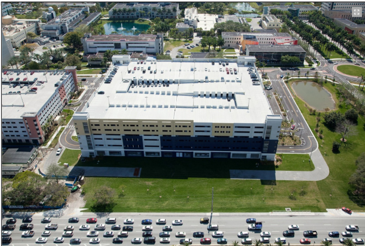
Figure 2-18 FIU PG-6 Aerial Image
