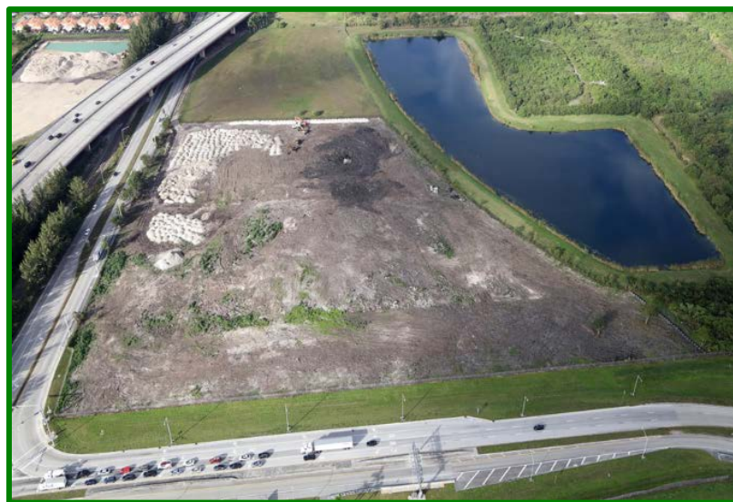
NORTH OF 12 TH STREET AND WEST OF HEFT – LOOKING WEST
