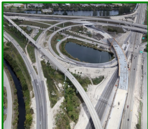
New flyover at SR 826/I-75 Interchange
