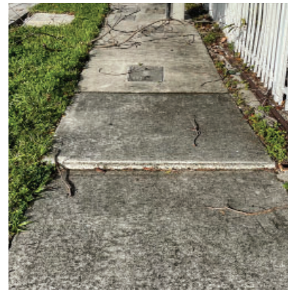
Damaged / Settled Sidewalk
