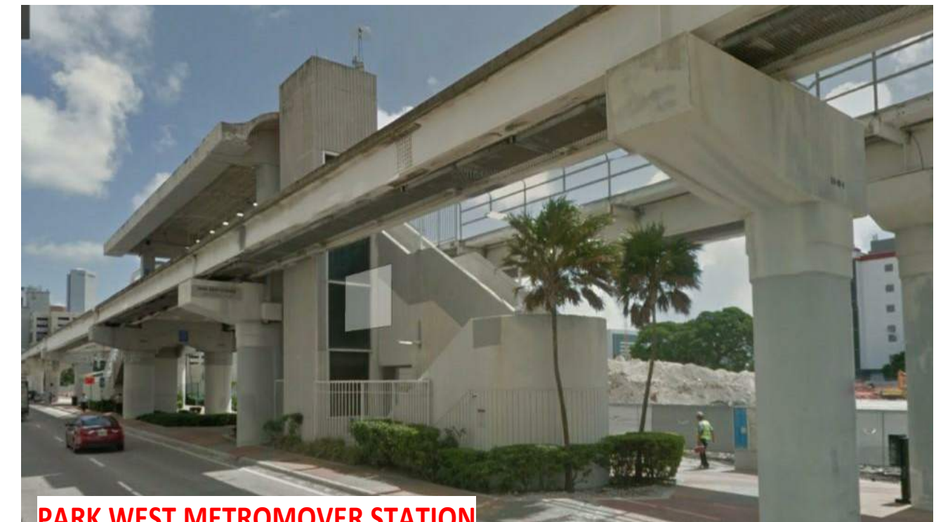
PARK WEST METROMOVER STATION SOUTH END CORNER OF NE 2nd AVE AND NE 8th STREET
